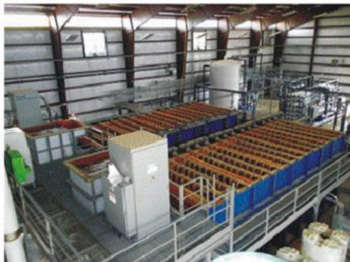
Twin train 500-gpm EC coupled with UF and RO
