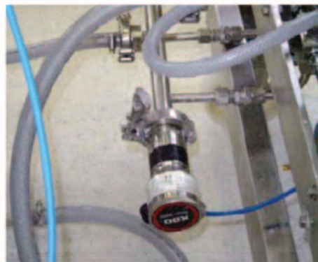
Figure 2. Installation of 9000 Series pressure transmitter.
