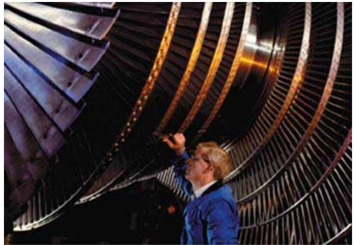
Fig. 1: Maintenance of a Hydrogen-cooled generator.
