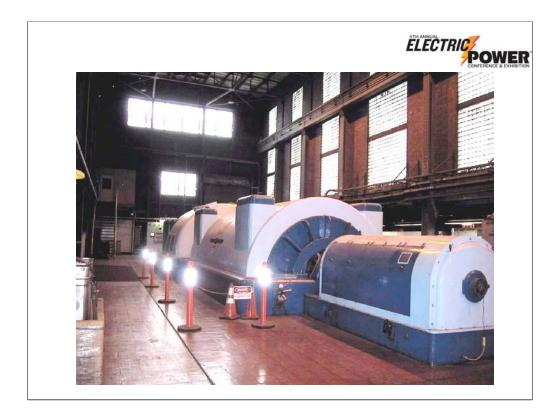
Hydrogen cooled generator – sealed cavity – recirculating pressurized hydrogen atmosphere
