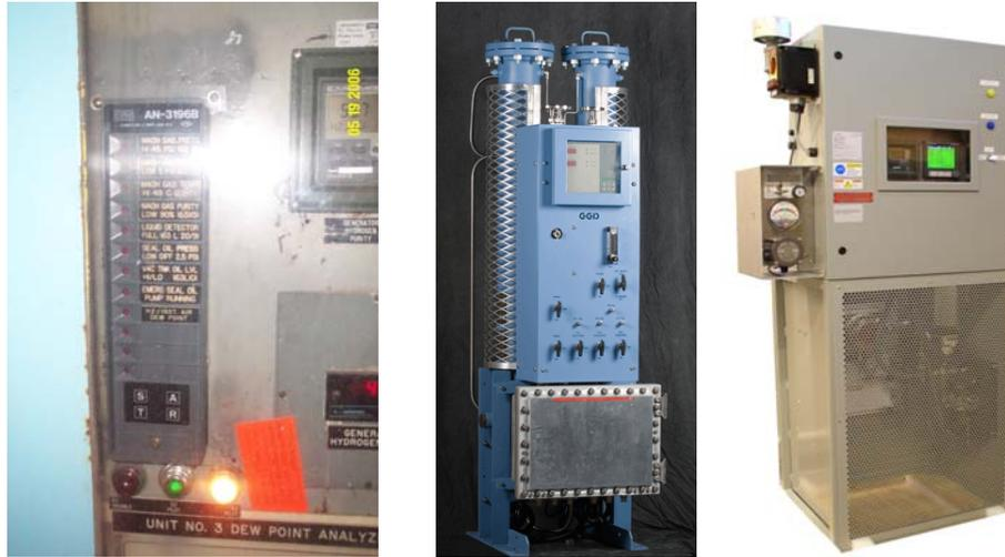
The dewpoint of the hydrogen in the generator casing can affect the lifetime of the generator windings. Wet hydrogen will reduce winding life due to corrosion. Wet hydrogen can be catastrophic in the case of 18/5 rings, susceptible to stress crack corrosion. You must keep dewpoint within manufacturer specs.
