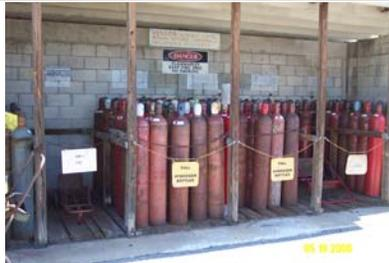
Technology choices on the hydrogen supply side of the generator: stored hydrogen or generated hydrogen. A certain amount of stored hydrogen is required for regas.
