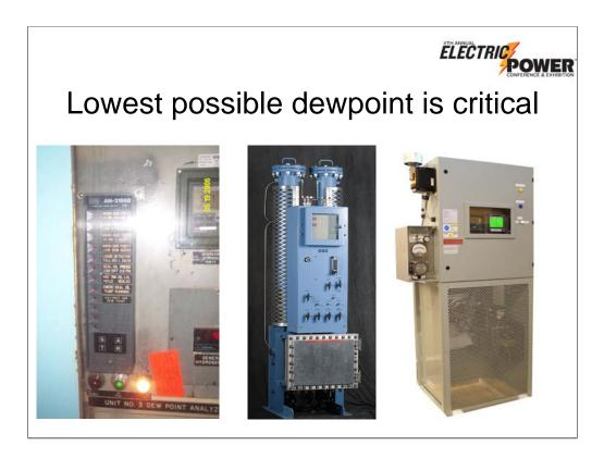
The dewpoint of the hydrogen in the generator casing can affect the lifetime of the generator windings. Wet hydrogen will reduce winding life due to corrosion. Wet hydrogen can be catastrophic in the case of 18/5 rings, susceptible to stress crack corrosion. You must keep dewpoint within manufacturer specs.
