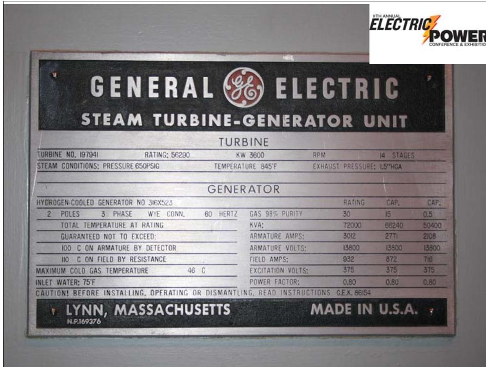
Note the manufacturer plate on your generator, and the guidelines in the user manuals. The gas in the generator casing must be kept at the manufacturer recommended purity in order to achieve the manufacturer commitment on heat rate. Note that the generator capability varies according to the gas pressure in the casing – if pressure is allowed to degrade – think Bleed & Feed – then the generator cannot deliver full capacity.
