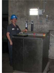
By making your own gas stored for regas, it is possible to entirely eliminate hydrogen deliveries. Self-generated backup/regas hydrogen at Luna Energy in NM and at Basin Electric in ND. Self-generating backup hydrogen is well-suited to plants that are geographically remote, or that have unique security requirements.
